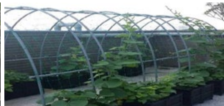
Community reformation - the construction of sky garden on roof (after reforming)
