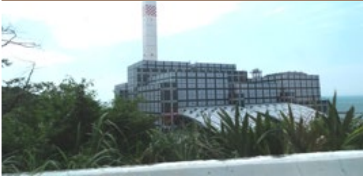
Picture of the Bali incineration plant
