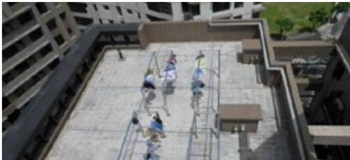
Community reformation - the installation of solar energy on roof (before reforming)
