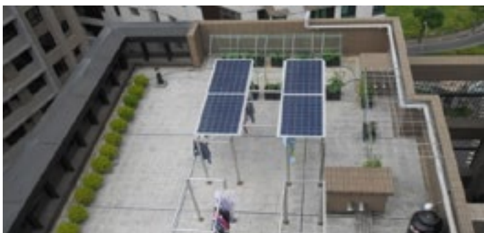
Community reformation - the installation of solar energy on roof (after reforming)
